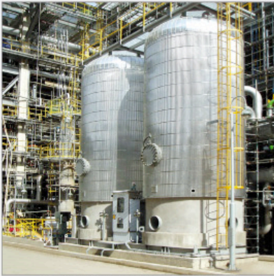
S-OIL N 2 RE-FINERY SYSTEM
